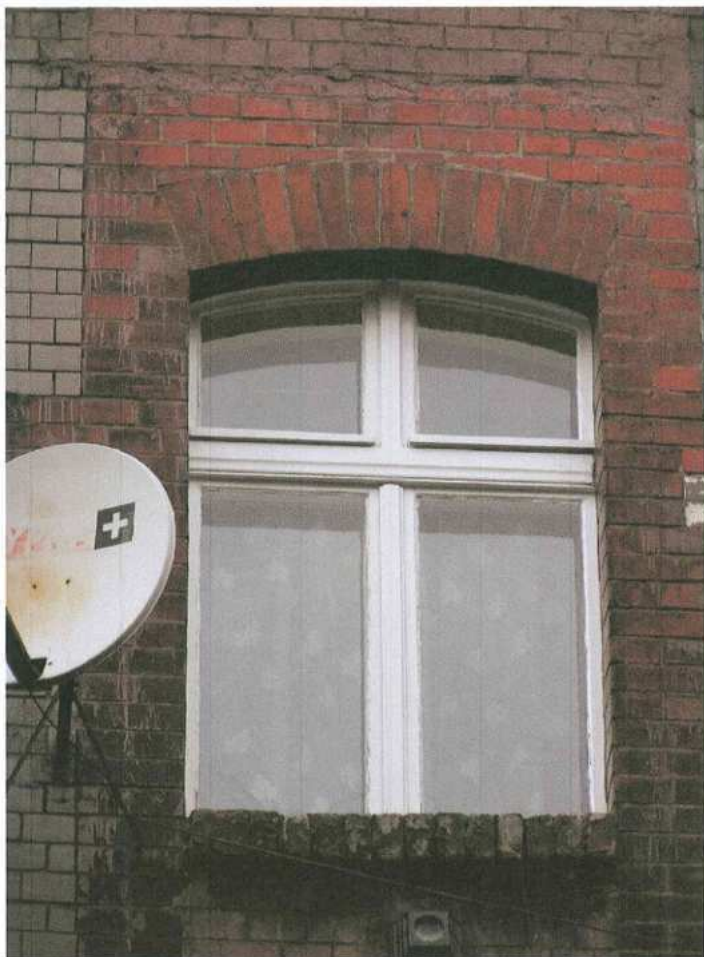
11.stolarka okienna w fasadzie
